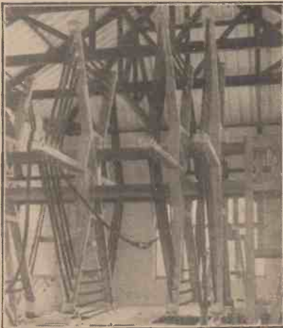
The primary inductance coil of the Rugby Station.
