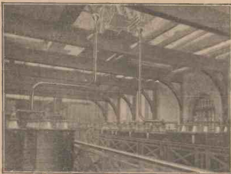
These condensors at the Rugby Station have a total capacity of 1.3 \mu\text{F} , and are mica-insulated.
